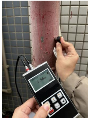
Post-Fireproof Coating Pipelines Measurement
