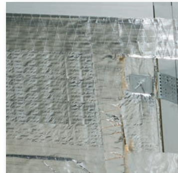
With aggressive adhesive and dead soft aluminum, 3M™ Foil Tape 3380 seals and secures seams and joints for long-term durability. UL 723 Listed for duct sealing and general repairs.
