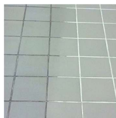
Clean Tile & Grout
