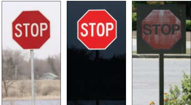
Signs that are MUTCD compliant provide clear guidance to drivers, day and night. Non-compliant signs do not command the same degree of attention and put property visitors at risk.
