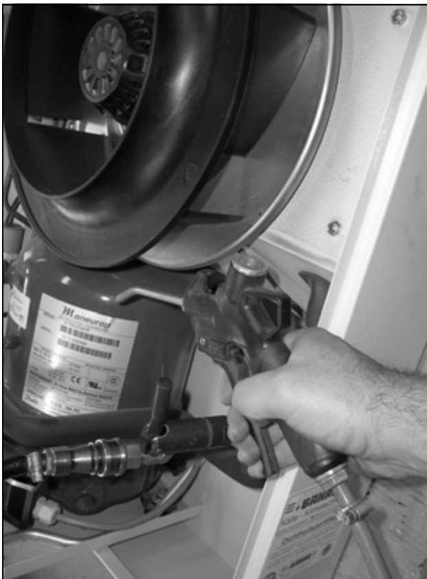
Fig. 56: Clean out the heat exchanger coil and compressor chamber using compressed air (2)
