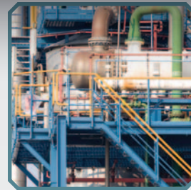
Structural Steel and Rails
