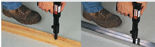
2" x 4" to concrete slab
