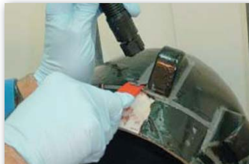
Edge Sealant Removal
